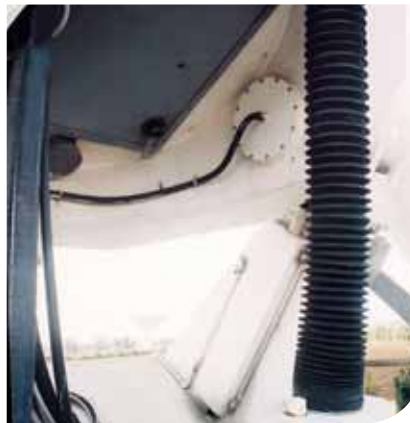
Bellows fitted to protect satellite dish screw jacks
